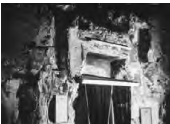
Fig. 10. The rectangular recess and the upper part of the apsidal niche.
